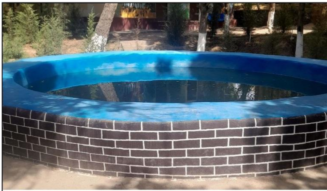
Rainwater harvesting reservoir
